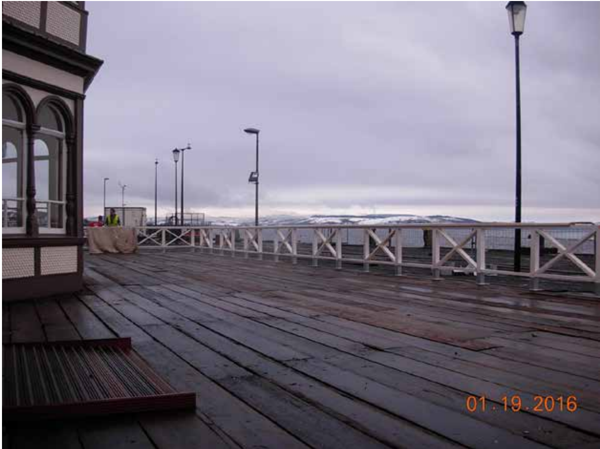
Pierhead – January 2016. Timber balustrade is being installed to demarcate the area that has been refurbished from the area which to be refurbished in Phase 2. The balustrade has been designed to the same specification and dimensions as the the original feature.
