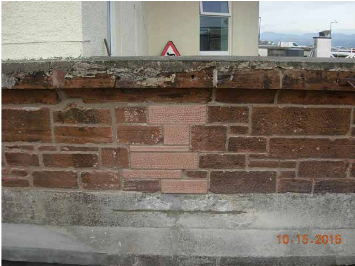
Retaining Wall to Harbourmasters Building – stonework repaired/replaced, repointed and concrete repaired
