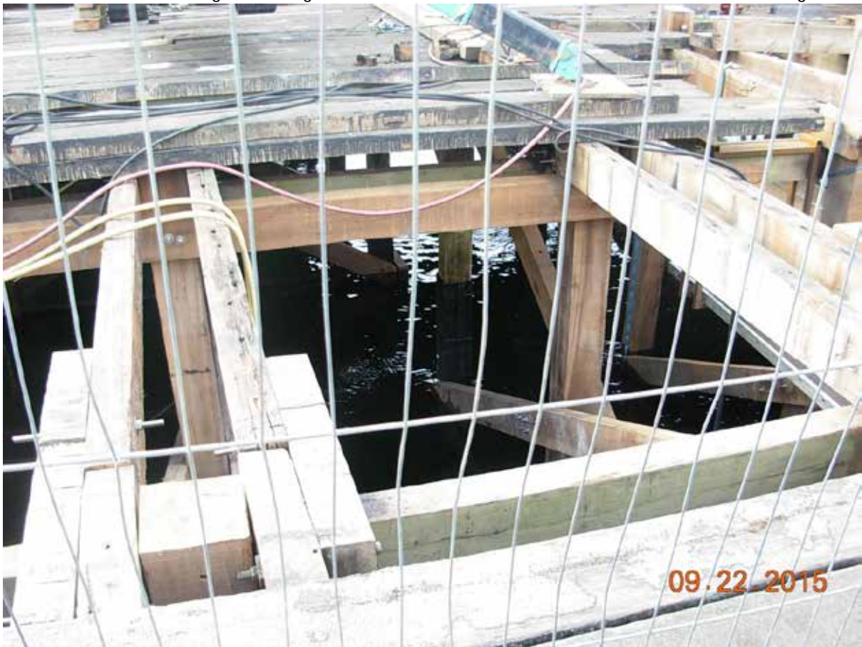
Structure of Pier – May 2014. Note longitudinal timber ties are missing to the foreground, diagonal timber braces are missing or no longer connected to the structure and timber columns are degraded
