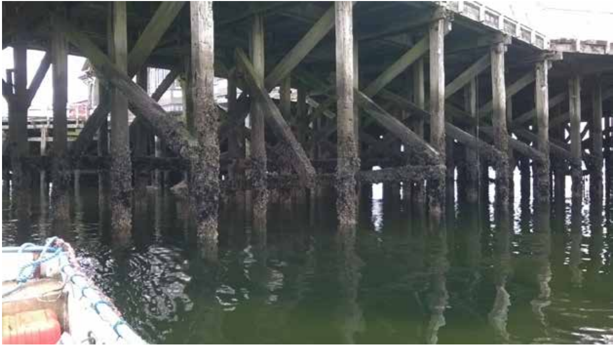
Structure of Pier – May 2014. Note longitudinal timber ties are missing to the foreground, diagonal timber braces are missing or no longer connected to the structure and timber columns are degraded
