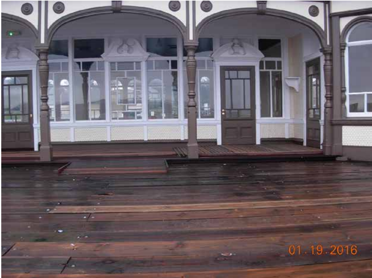
Waiting Room – January 2016. Veranda decking has been replaced and access ramps have been created to allow wheelchair access into the waiting room building. Decking is yellow balau and includes a resin/aggregate anti-slip application to the ramps and platform areas. Area of main decking in the foreground is awaiting application of Deckcoat anti-slip treatment.
